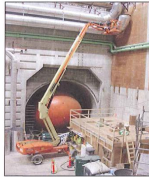
Man lift in use to install duct.
